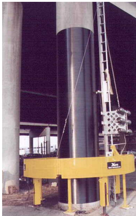
FIGURE 4 INSTALLATION OF CARBON WRAPS USING ROBO-WRAPPER I TM
