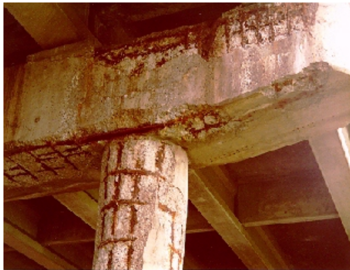
FIGURE 3 CORRODED CAP BEAM & COLUMN, HOOP & VERTICAL STEEL WEAKENED
