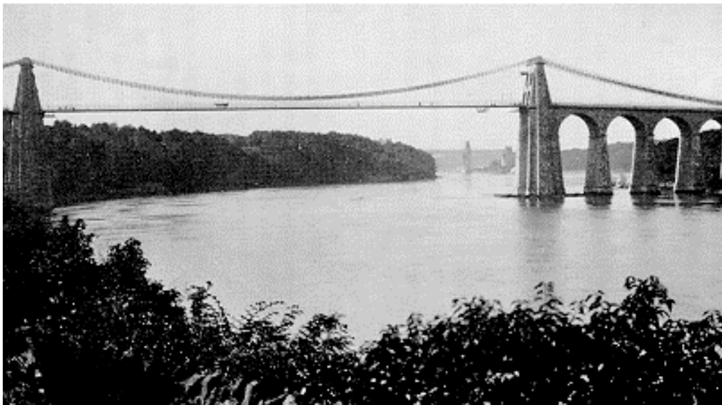
FIGURE 2 PHOTOGRAPH OF FIRST MODERN SUSPENSION BRIDGE DESIGNED BY TELFORD (1826)
