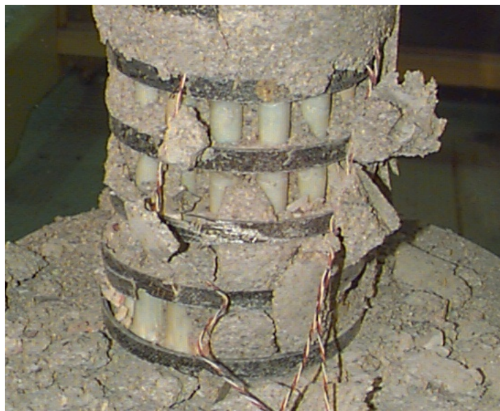
FIGURE 27 CONTINUATION OF END FAILURE FOR 1 ST GENERATION
