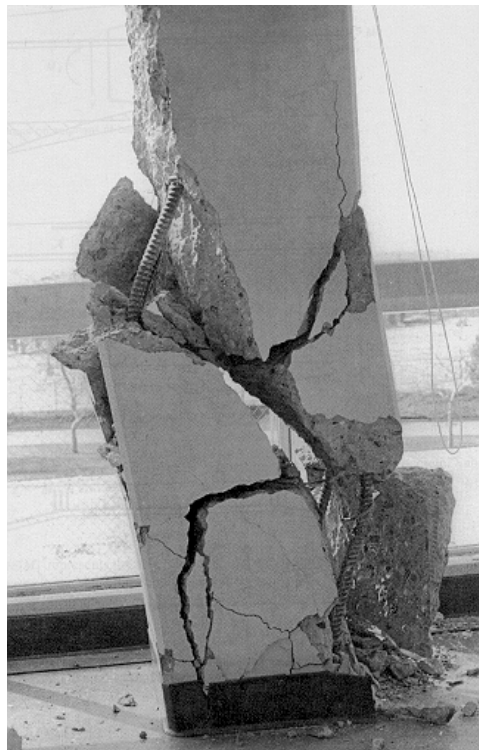
FIGURE 40 PHOTOGRAPH OF SHEAR FAILURE IN REINFORCED COLUMN
